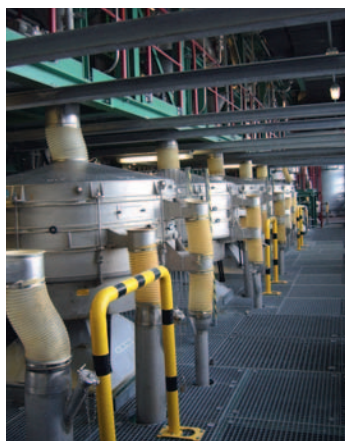
Establishing connections to tumbler screening systems
